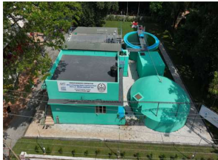
360 KLD STP at General Hospital, Thrissur
